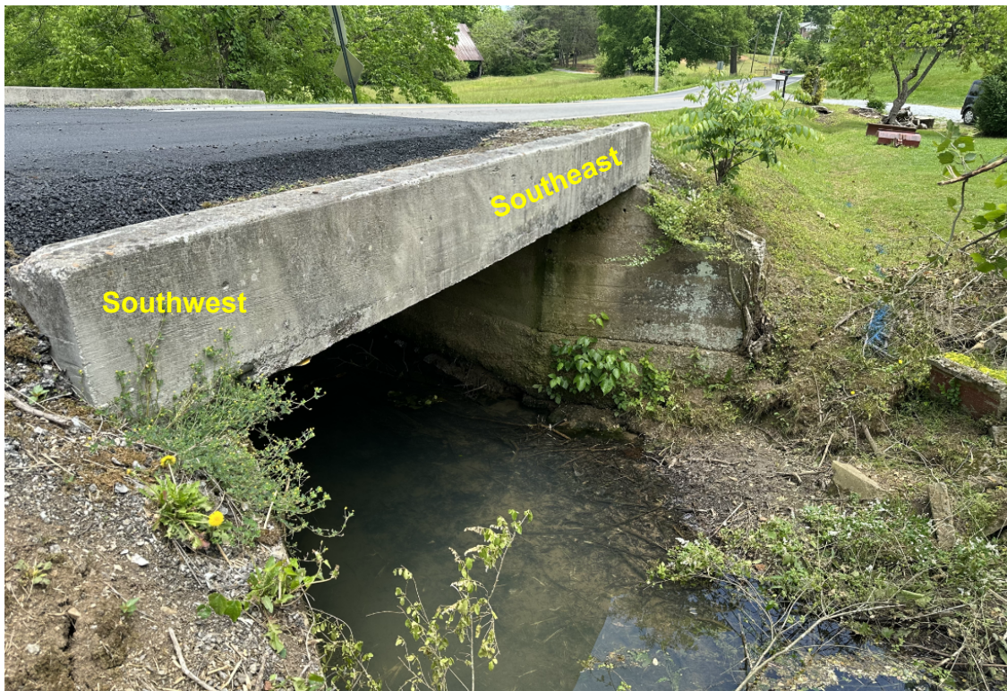
Figure 3 – Downstream bridge conditions as of 5/18/23
