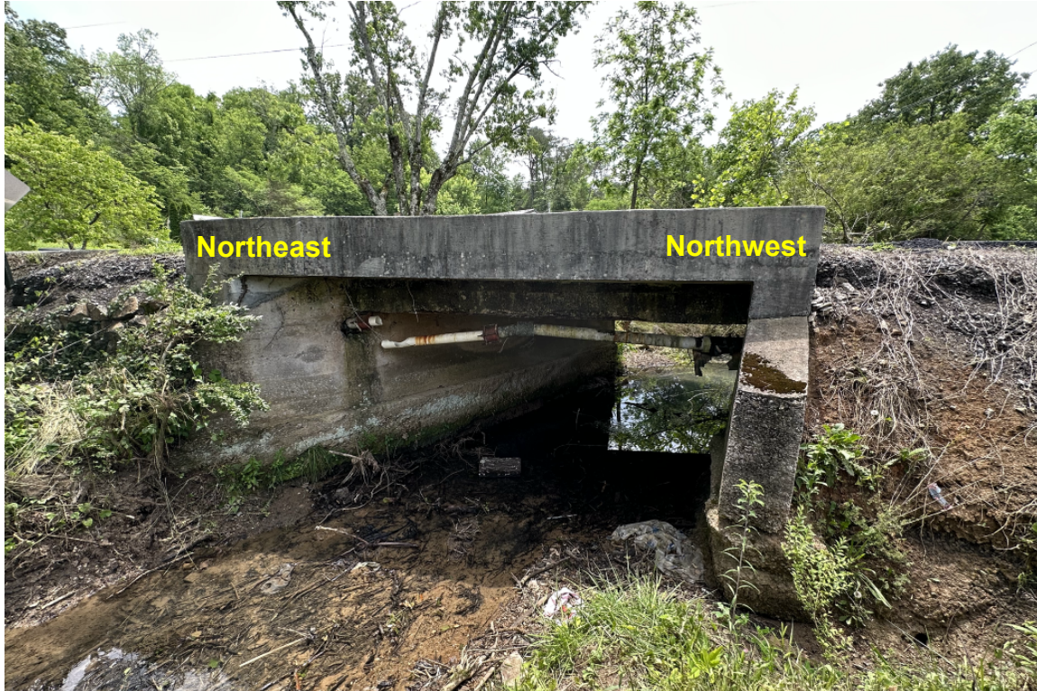
Figure 2 – Upstream bridge conditions as of 5/18/23
