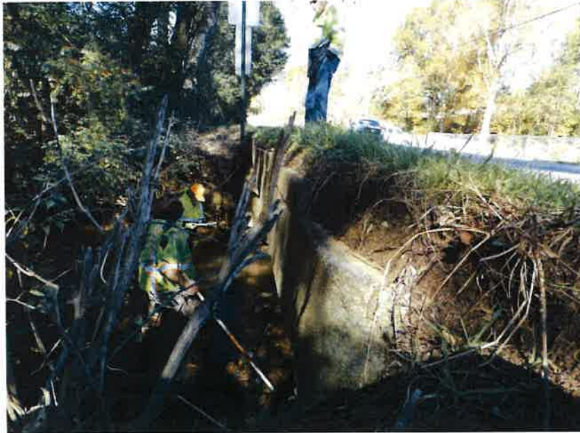
ROTATION OF RIGHT SIDE HEADWALL
