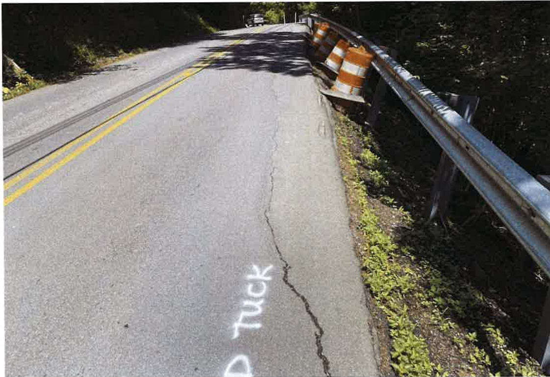
Figure 2 – Existing conditions along Old Tuckaleechee Road
